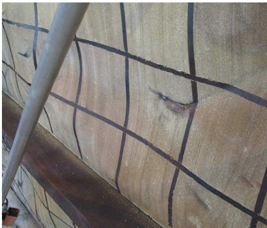
Fig. 19. Cracks in the steel plate.
