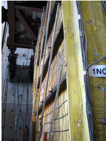
Fig. 18. First-story steel plate buckling.
